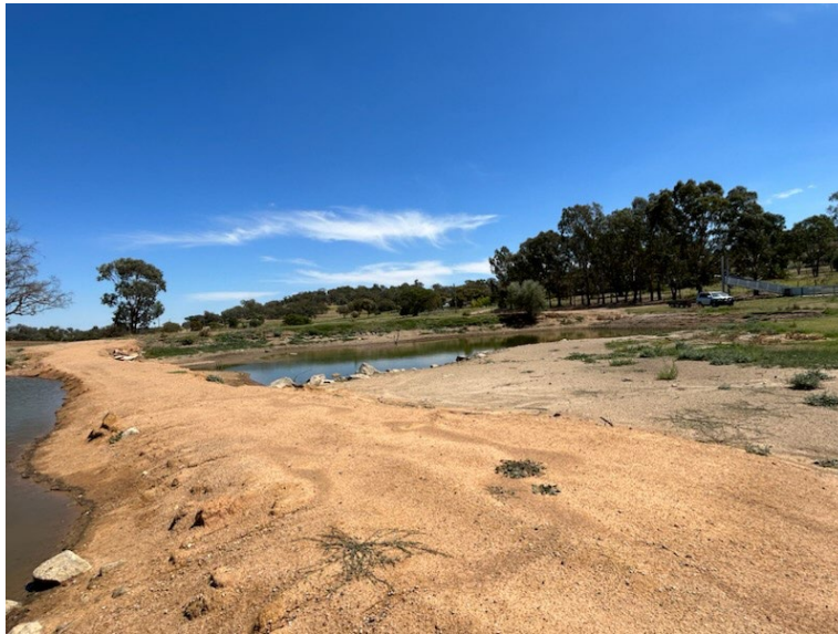
Image showing the current retaining bank on site (large dam to left) – stockyards to the top right of image. The small dam to the right will be back filled and vegetated.
